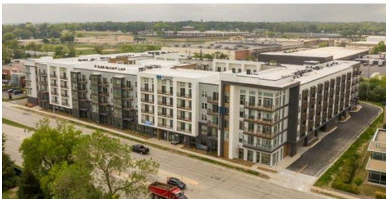
2929 North Mayfair Road New 258 Unit Apartment Building
